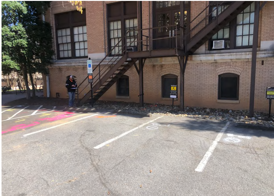
Figure 1-1 – Existing Site Conditions on March 12, 2024
